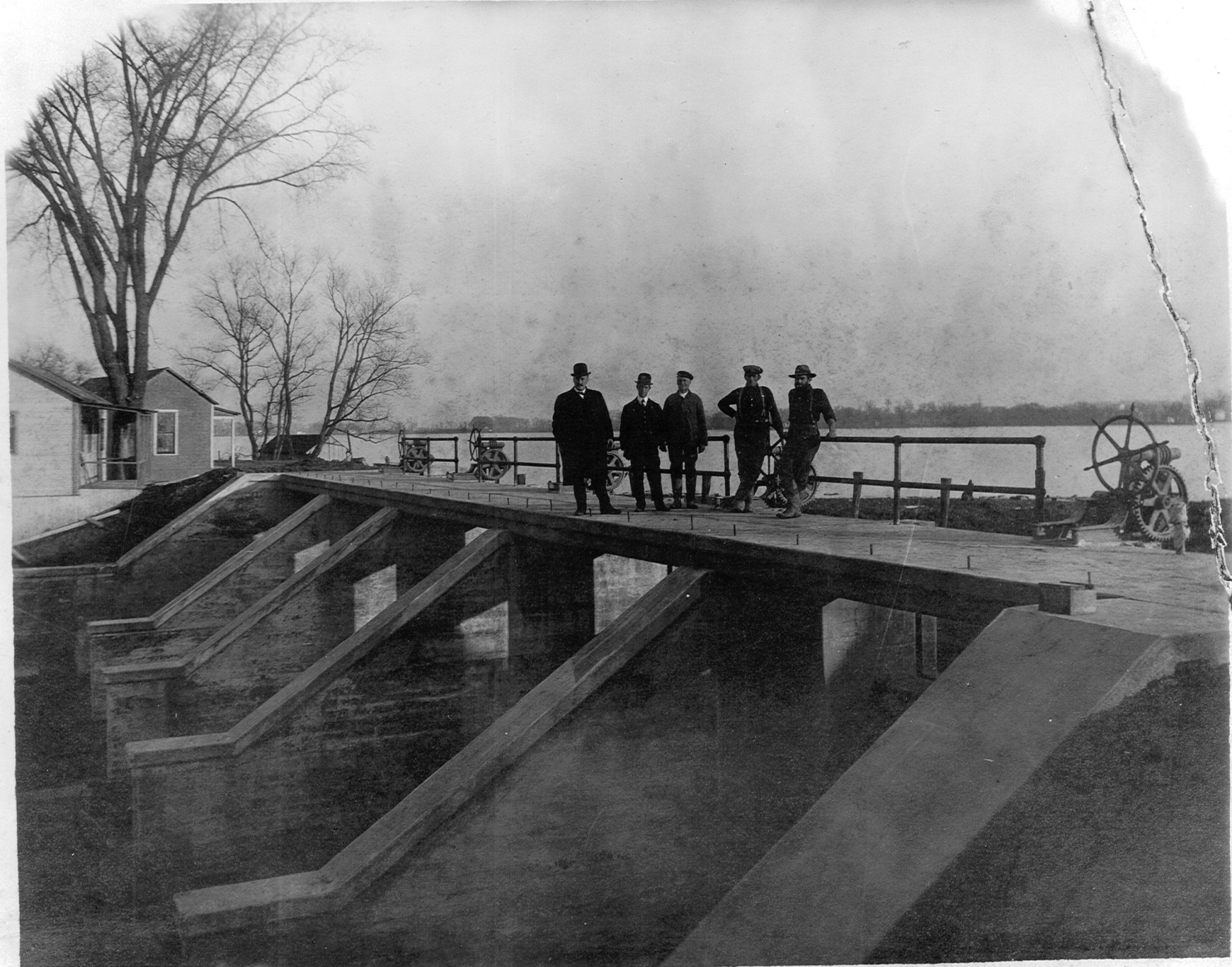
Completion of Kinnear Bros. Contractors of Buckeye Lake Waste Weir Dam to H. H. Rosebraugh —
