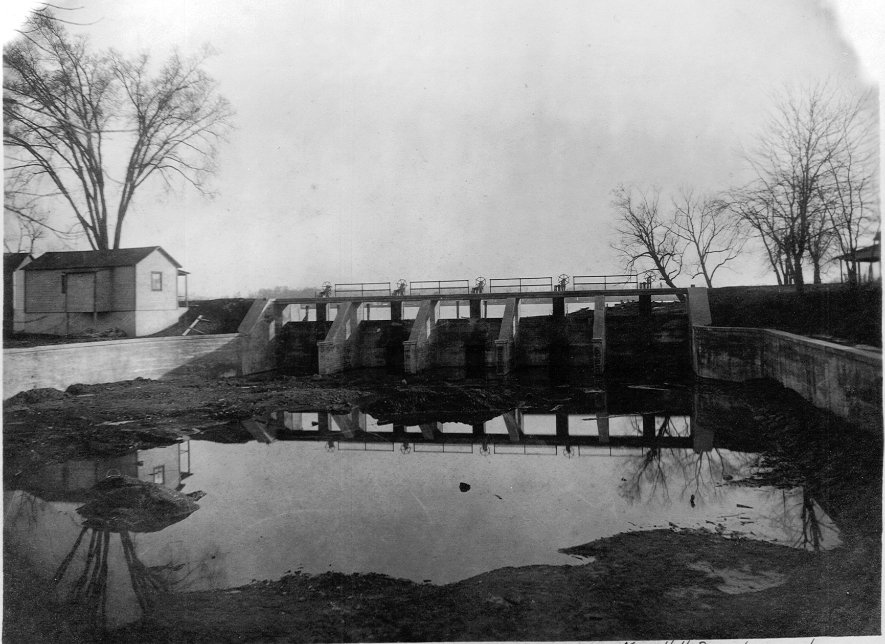
Completed by Kinross Bros Contractors of Buckeye Lake Waste Weir Dam to Mrs. H. H. Rosebraugh—
