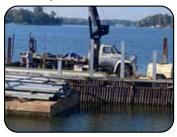
The work on the front basin continues. We have now completely back-filled behind the new sea wall. We have started the process of driving I-beams for the new pier on the west side of the island as well as starting to install the
